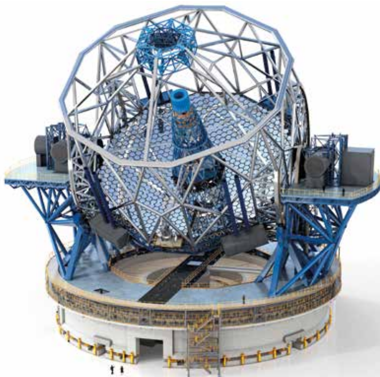
2 The inner structure of the ELT, showing the segmented primary mirror. (Courtesy: ESO/Dorling Kindersley)
