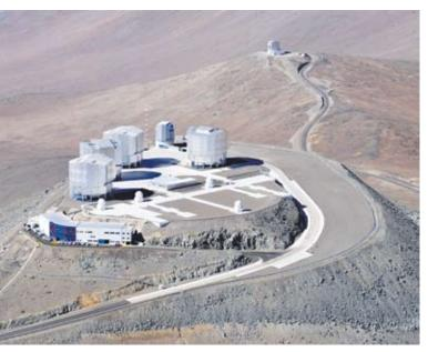
Figure 1. ESO site on Cerro Paranal. The VLTI is formed by four unit telescopes with main mirrors of 8.2 m diameter (large buildings) and four movable 1.8 m diameter auxiliary telescopes (small domed buildings). (Picture: ESO)
