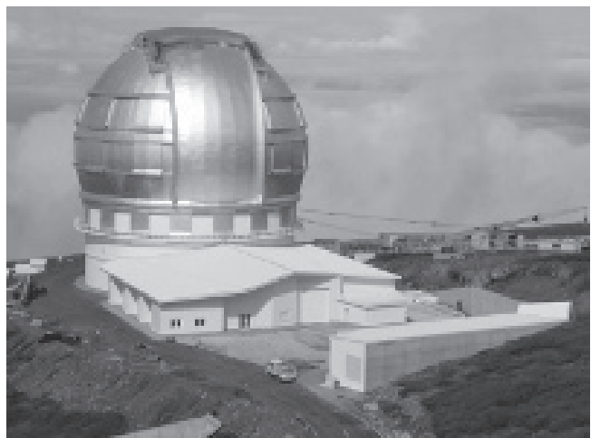
Figure 1. Grand Telescopio de Canarias under construction.
