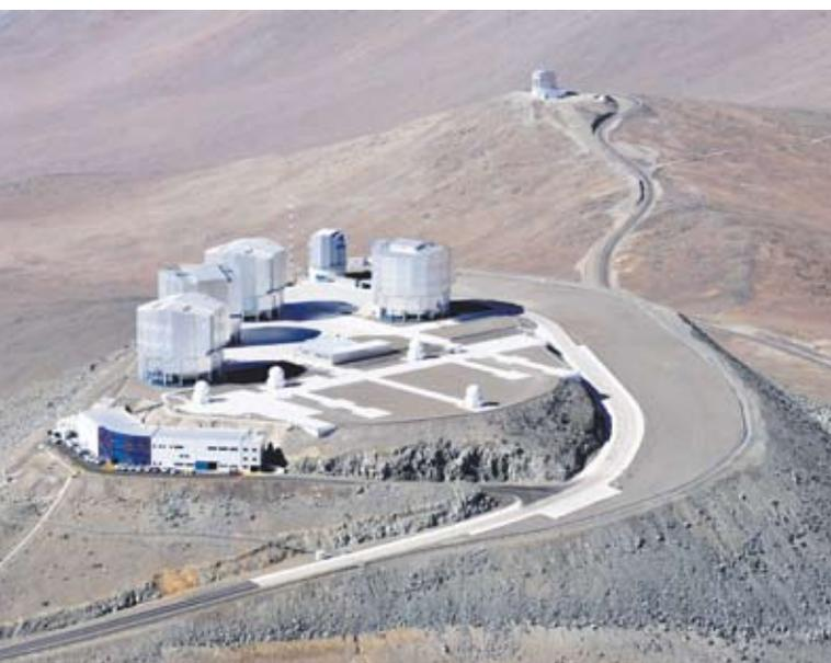
Figure 1. ESO site on Cerro Paranal. The VLTI is formed by four unit telescopes with main mirrors of 8.2 m diameter (large buildings) and four movable 1.8 m diameter auxiliary telescopes (small domed buildings). (Picture: ESO)
